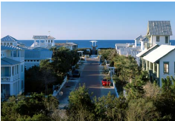
The axis, architectural features, and varied rooflines and of this street in Seaside, Florida create a place that feels unique and has set a high standard for TND to follow.
