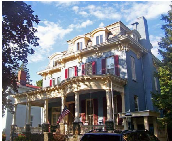
The Chichester House on Fair Street shows the importance of the front porch in Kingston's traditional architecture.
